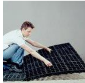
STEP 2 LAYOUT AND ALIGN BY ROW
